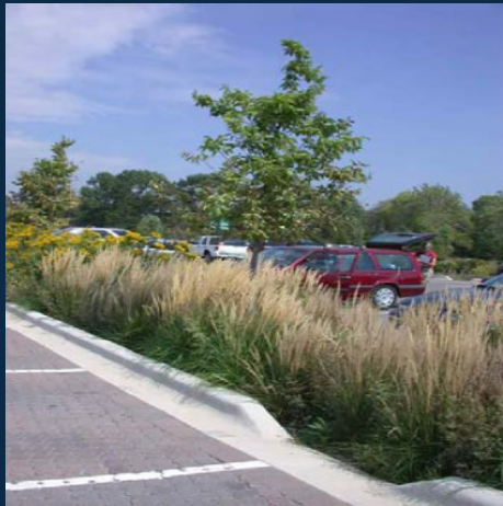
Curbing with depressed turnout for drainage
