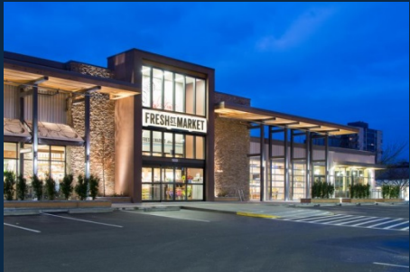
Utilization of stone and architectural metal panels as façade materials.
