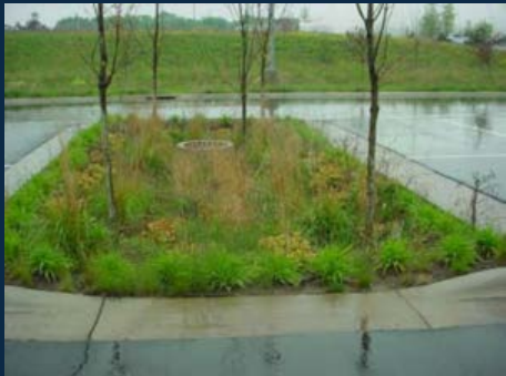
Parking island with ribbon curb for use as storm water BMP / rain garden
