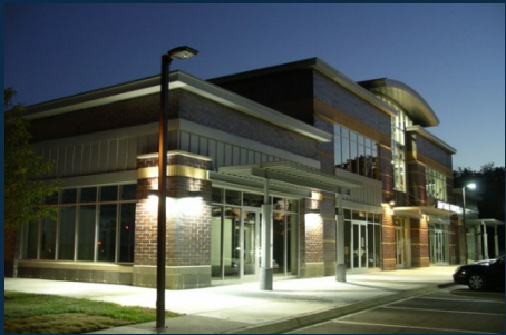
Utilization of brick, metal panels and cement board faux wood banding as façade materials
