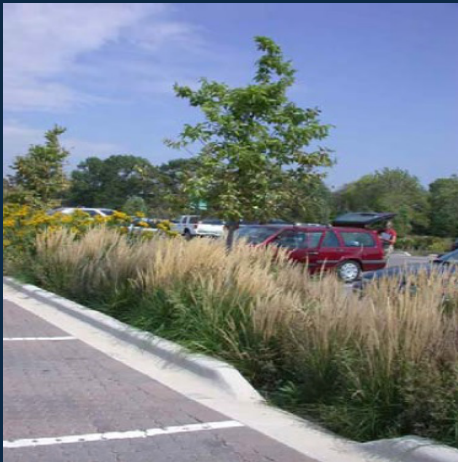
Curbing with depressed turnout for drainage
