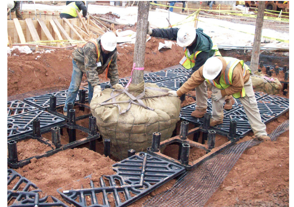
Tree Well Construction
