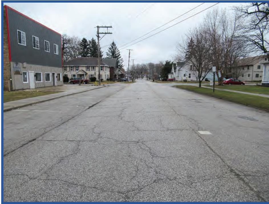
Photo 9: Looking north along Tipton Street towards Grove Street
