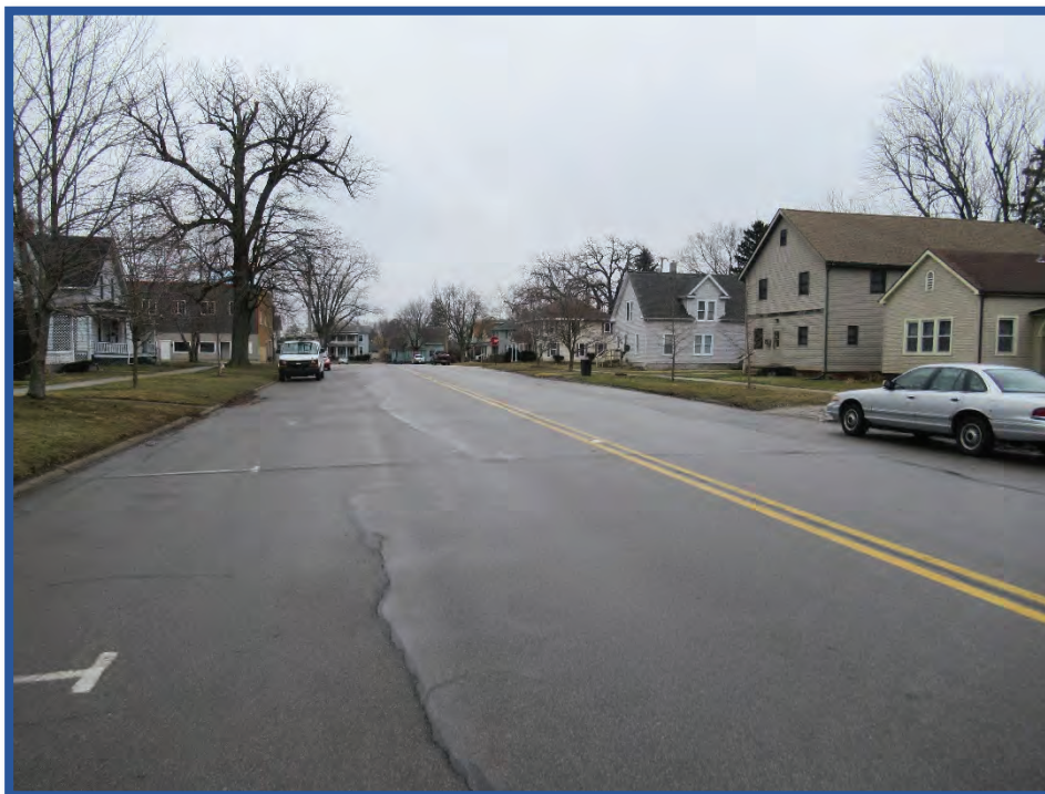
Photo 10: Looking east along Grove Street towards Tipton Street
