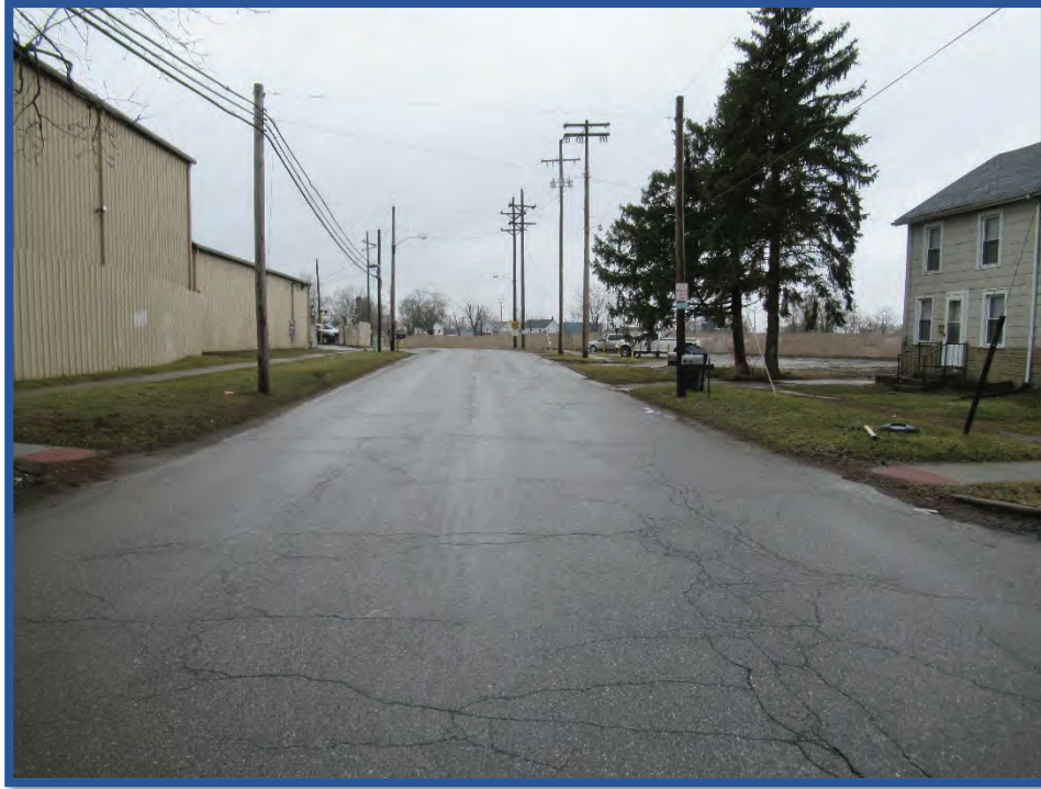
Photo 11: Looking south along Tipton Street from Furnace Street
