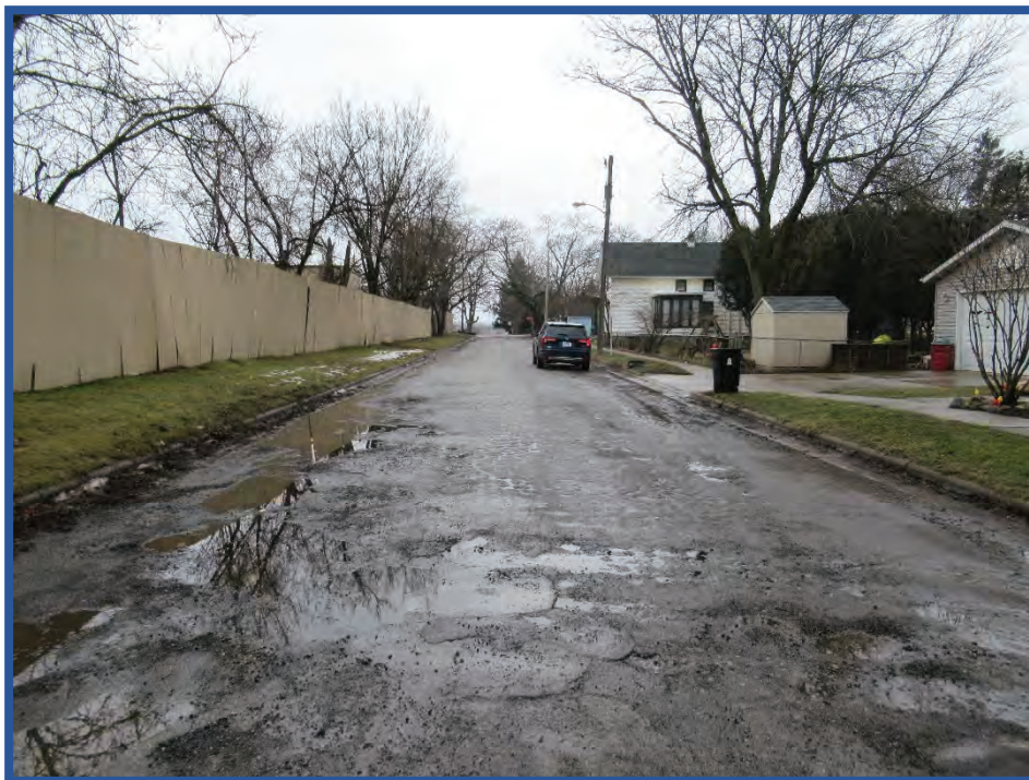
Photo 14: Looking west along Furnace Street from Pulaski Street
